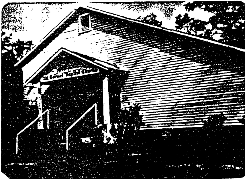
Building of 1905. As it looked in 1954.
