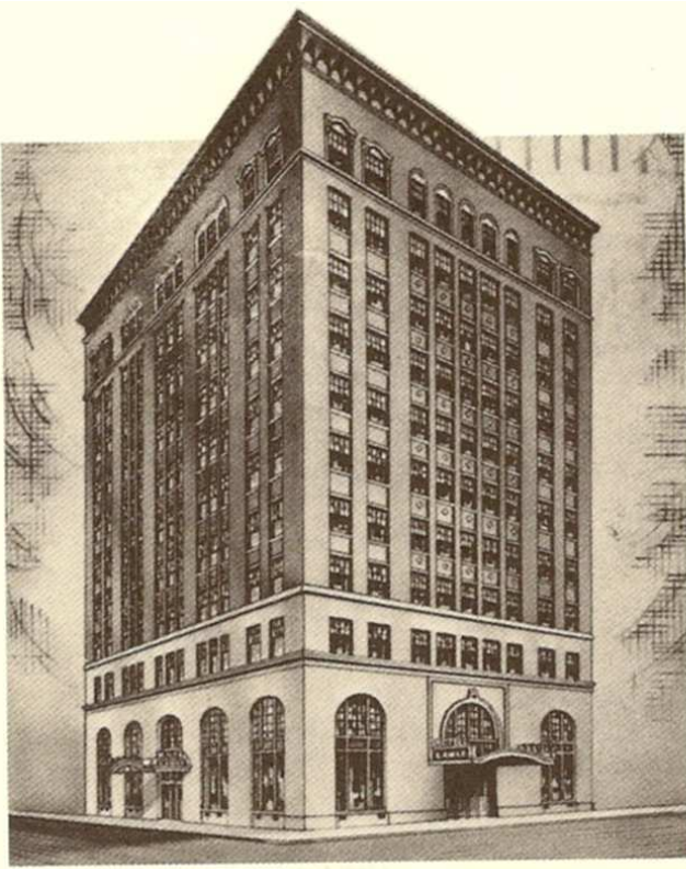
Hotel Lamar, now houses Lauderdale County Department of Archives and History
